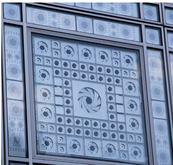
Figure 2: Jean Nouvel's Institut du Monde Arabe's mechanical iris system. Through an array of similar systems, a dynamic change happens as environmental conditions change.
